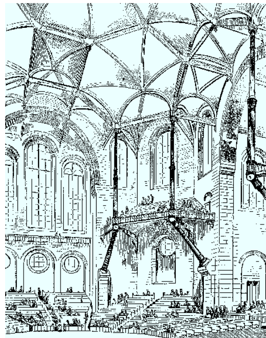
Fig 3: A sketch of a concert hall of brick and cast iron by Viollet-le-Duc [22]
